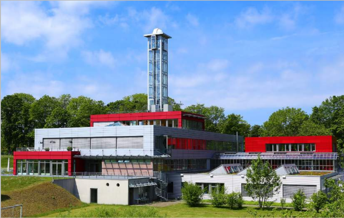
Pulverhaus view from tailings
